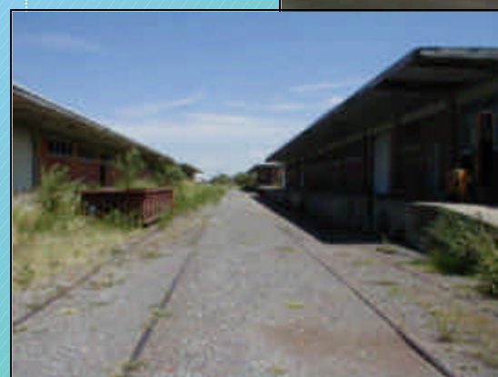
Rail Spur Adjacent to Vacant Warehouses
